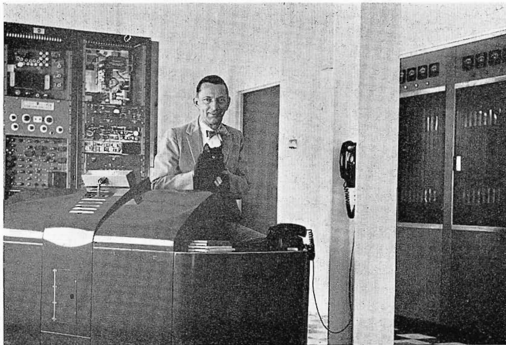
FIG. 2. Author Dean Spires, transmitter supervisor in control room of TT-10AH TV Transmitter, note official station mascot, "Buford."
