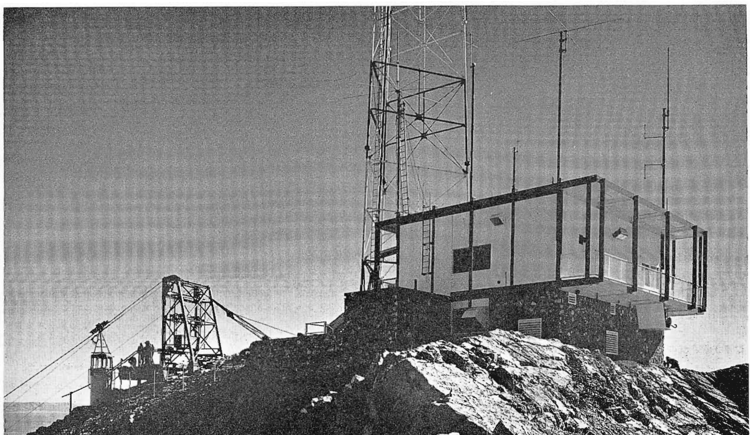
FIG. 3. The peak of the mountain was blasted off to provide room for the building and tower.
